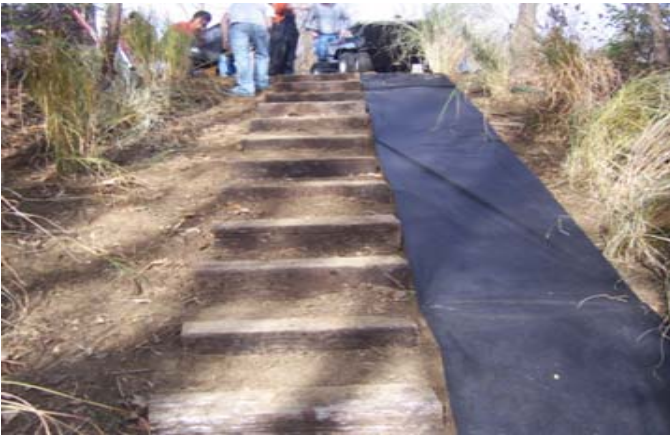
Ornamental grass and weed netting installation.
