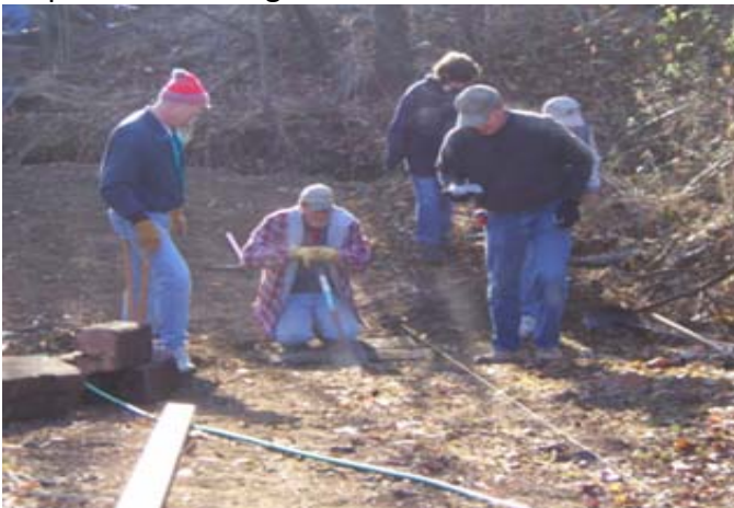
Step installation – garden side.
