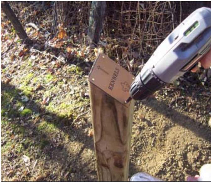
Directional Signage installation.
