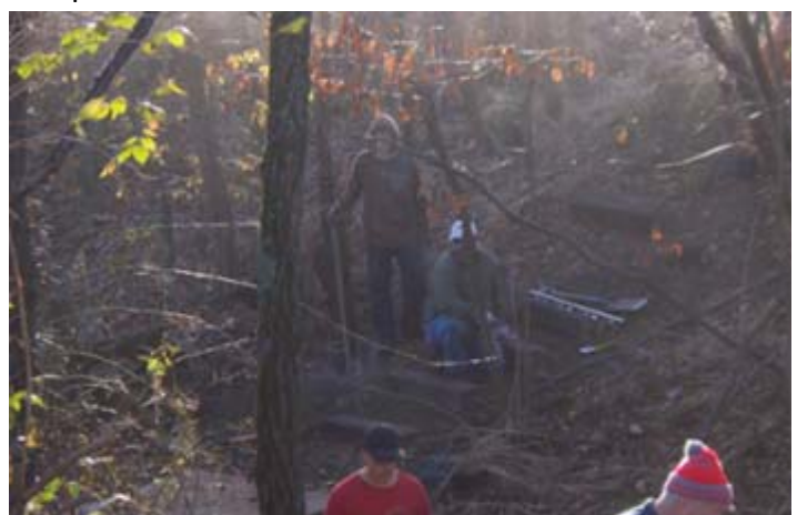
Step installation – kennel side.
