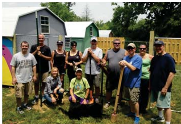
Board Members and volunteers put up fencing for new play yards for the dogs!
